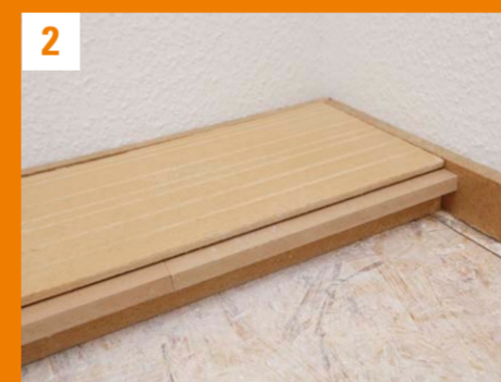
2 AGEPAN® TEP passgenau und fugendicht verlegen AGEPAN® TEP must be exactly laid with seamless joints
